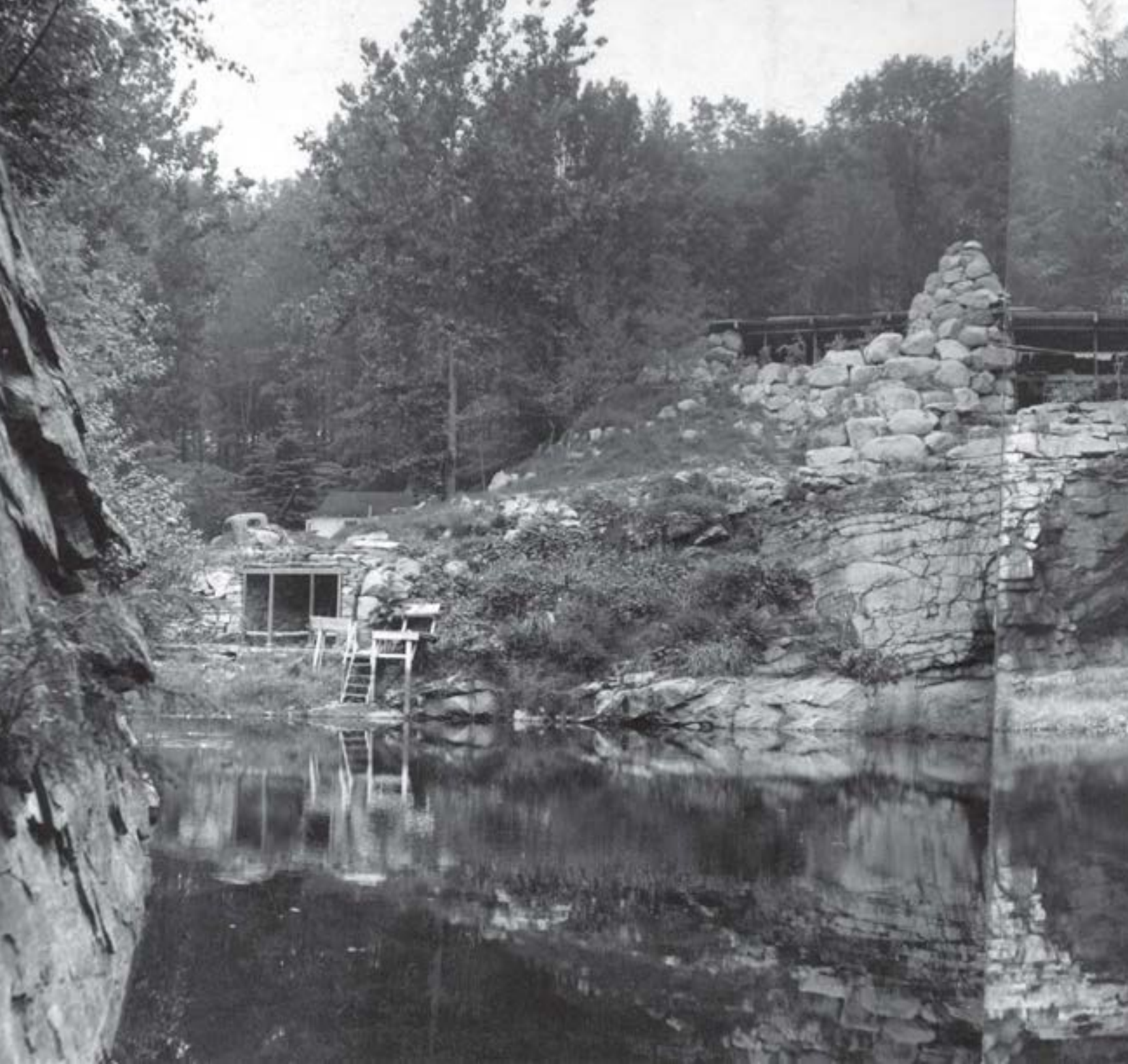
An old photo illustrates Dragon Rock under construction. Photo courtesy of Manitoga/The Russel Wright Design Center
